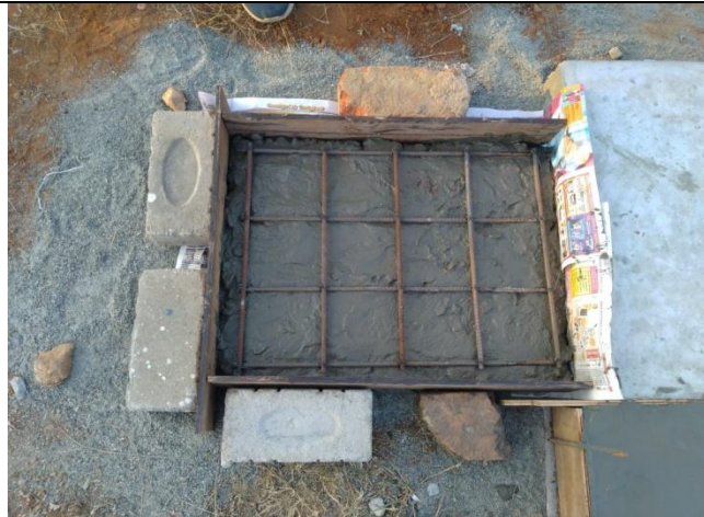
Fig 3.2 Formwork of slab casting with reinforcement
