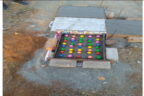
Fig. 3.3 Insertion of plastic balls (25) in slab casting
