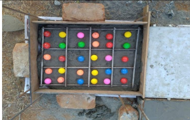
Fig. 3.4 Insertion of plastic balls (30) in slab casting
