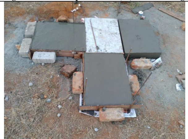
Fig. 3.7 Completion of Bubbled slab casting
