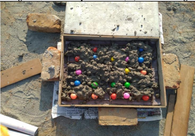
Fig. 3.6 Pouring concrete in plastic balls (25) slab casting
