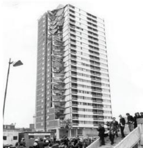
Fig. 1 Ronan Point Building after Collapse
