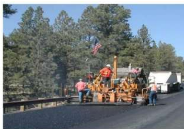
Fig -6: Rubberised bitumen construction
