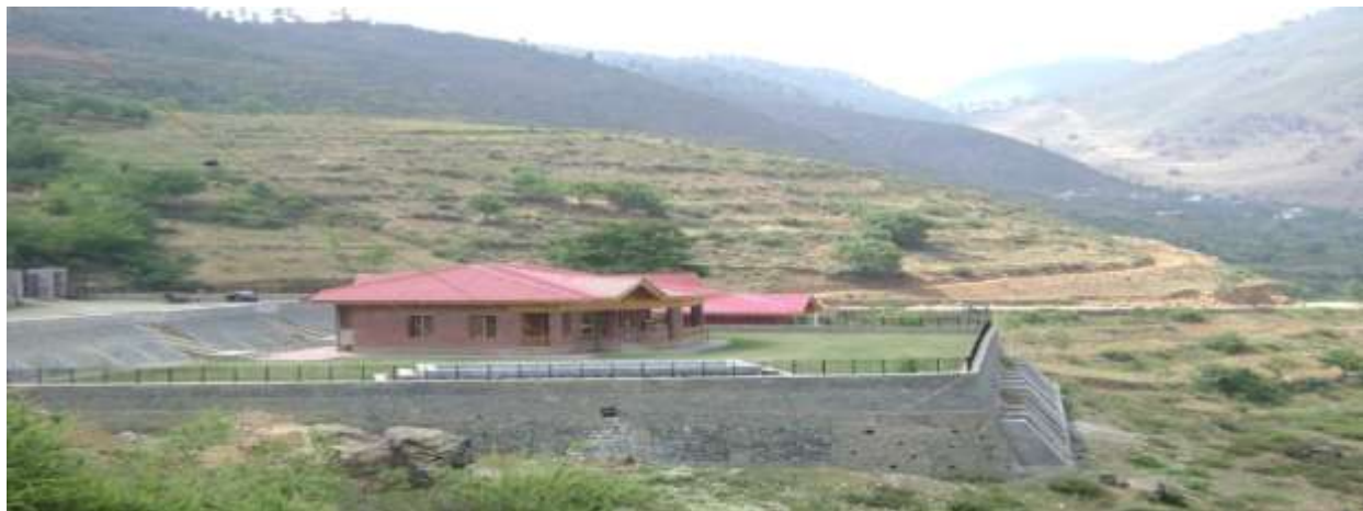
Photo 1.5 Encroachment of Tourism Department along the lake catchment which has led to deforestation and unstable hill slopes
