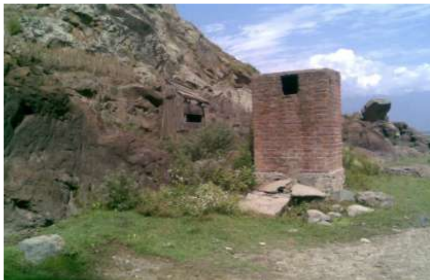
Photo 1.7 Lavatories with open drains entering the lake area
