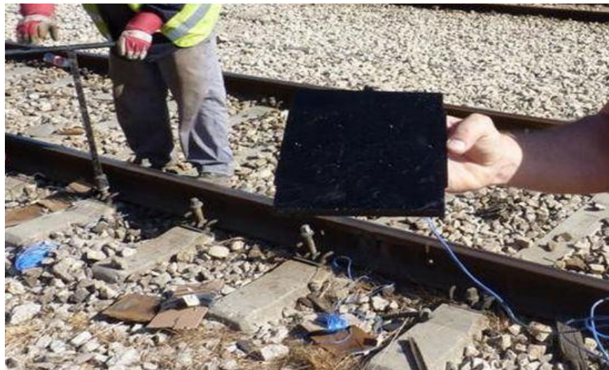
Fig. 2. Working construction in Delhi Metro Rail Track for Generation of Power [5]
