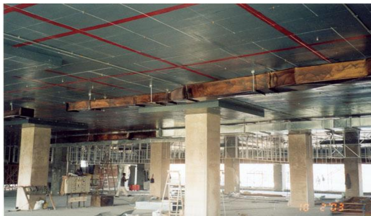
Fig.3 Flexibility in providing AC ducts
