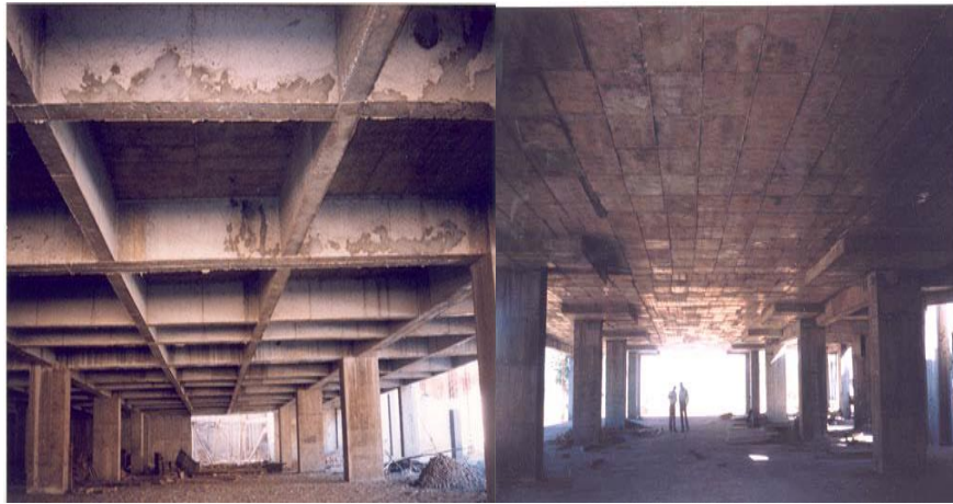
Fig.1 Conventional floor slab system with beam depth
