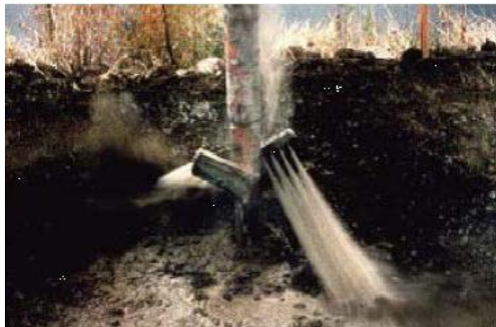
Parts of wet mixing tool showing injection of slurry into the soil
