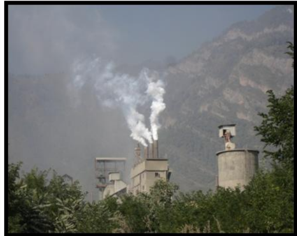
Dust and Gas Emissions from Khrew, Jammu and Kashmir, India (JK Cements)
