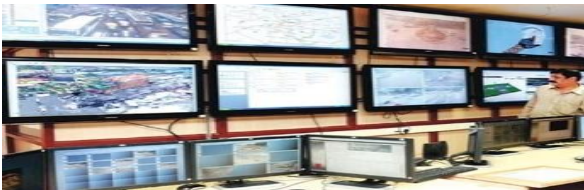
Fig1. 4 Bangalore Traffic Control Room
