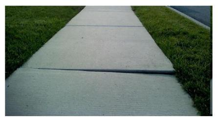
Figure. 5: Uneven Leveling of Concrete Slab
