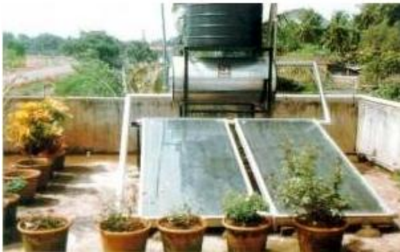
Fig: 4 Solar water heating system (SWH)
