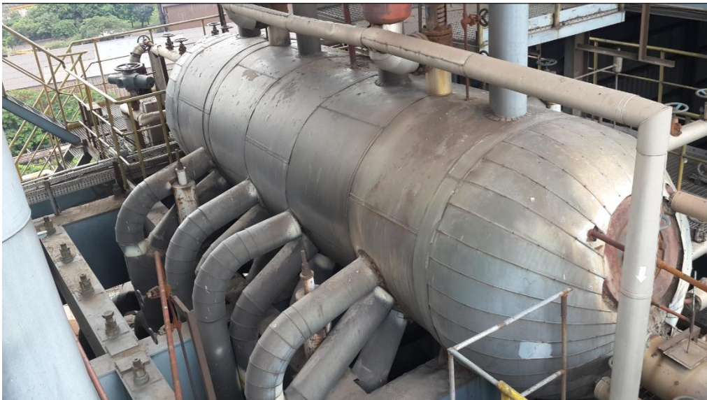
Fig. 1130 TPH CFBC Boiler Steam drum (Company: - BMM ISPAT LTD)
