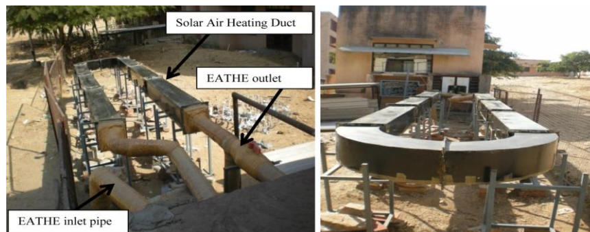
Fig.2. EATHE coupled with solar heating duct
