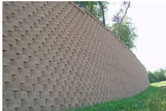
Fig.2 Segmental Retaining Wall
