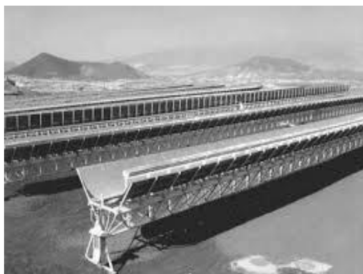
Figure.5: line Focus Parabolic Reflective Trough Concentrator
