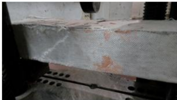
Fig. 3: Failed beam S1 after testing
