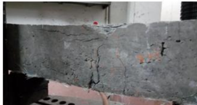
Fig. 14: Failed beam BF5 after testing
