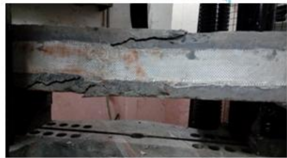
Fig. 8: Failed beam BS5 after testing
