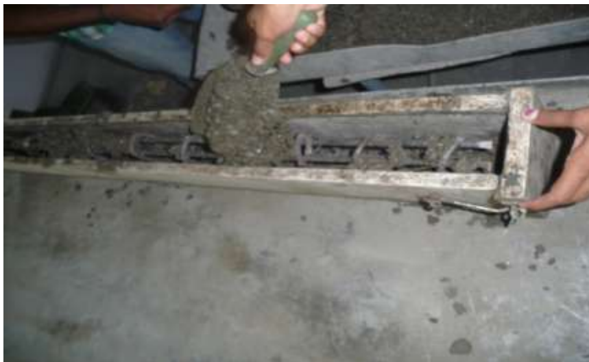
Fig.2. Casting of Reinforced Prototype Beam with MRFC
