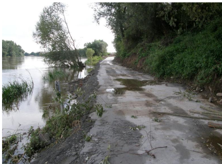
Figure 8: Flooding of base layer of still unfinished cycle paths from CCB during flooding (ČEZ a.s., 2013)
