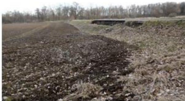
a) the greatest of the many failures of downstream face of the levees in the length of approximately 25 m
