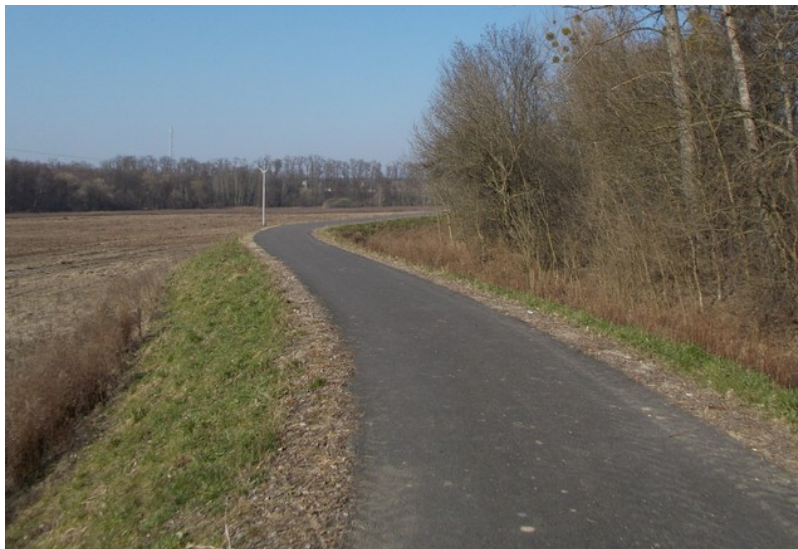
Figure 2: Levee with asphalt bicycle trail near the village Rohatec in the Hodonín
