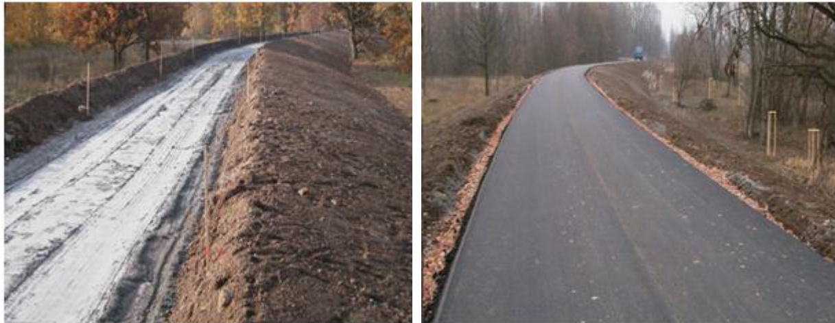
a) levee during construction
