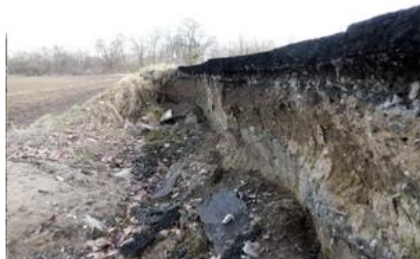
c) detail of exposed interior of the levee, including layers from fly ash stabilizer
