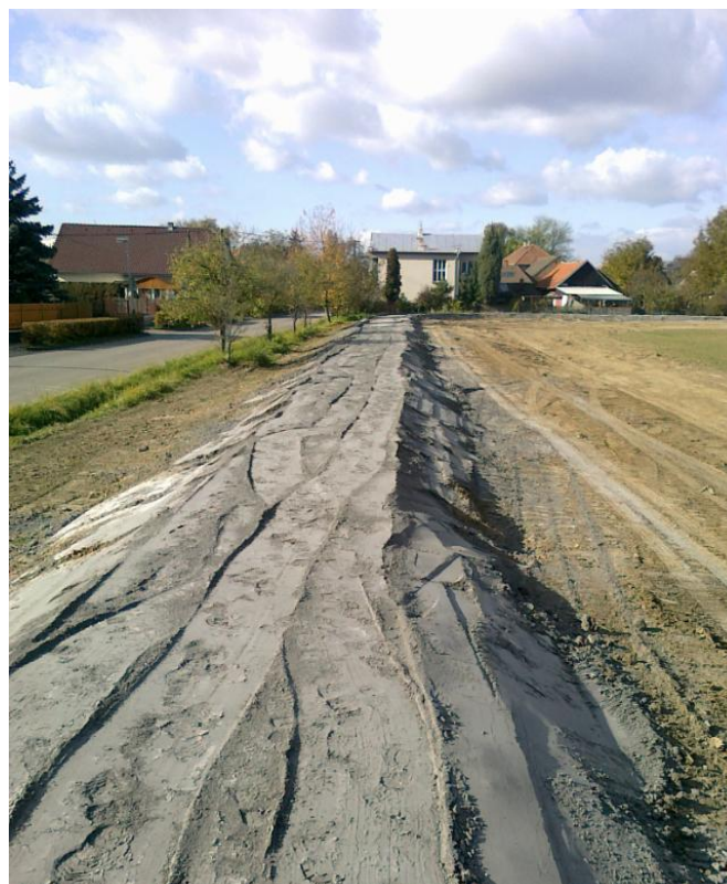
Figure 5: Vrды - Construction of Levee Using CCB (Power Plant Opatovice, 2014)
