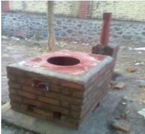
Figure 1. Photo of Jaggery Furnace
