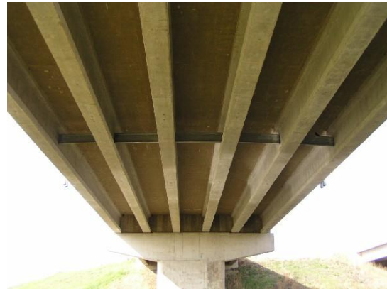
(b) Bottom view (center span and west pier)
