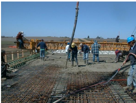
(c) 'MMFX bridge' deck concrete placement
