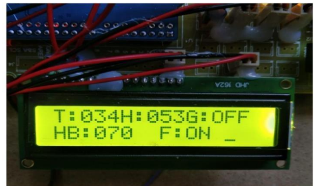
Fig 4: Smart safety sewage using IoT
