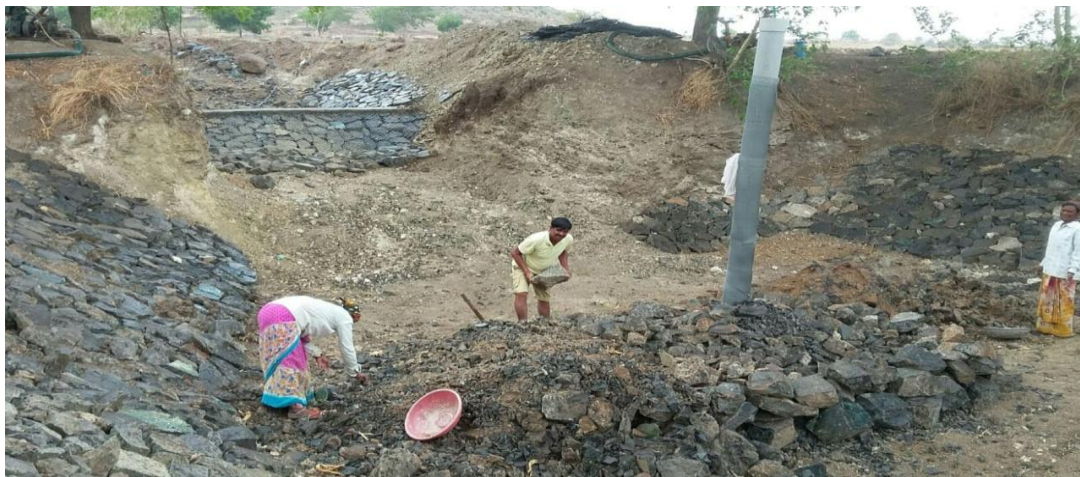
Image No. 3 –Construction of filtration Chamber
