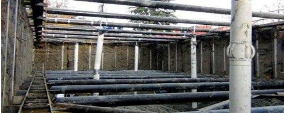
Fig. 2 – Bracing excavation method
