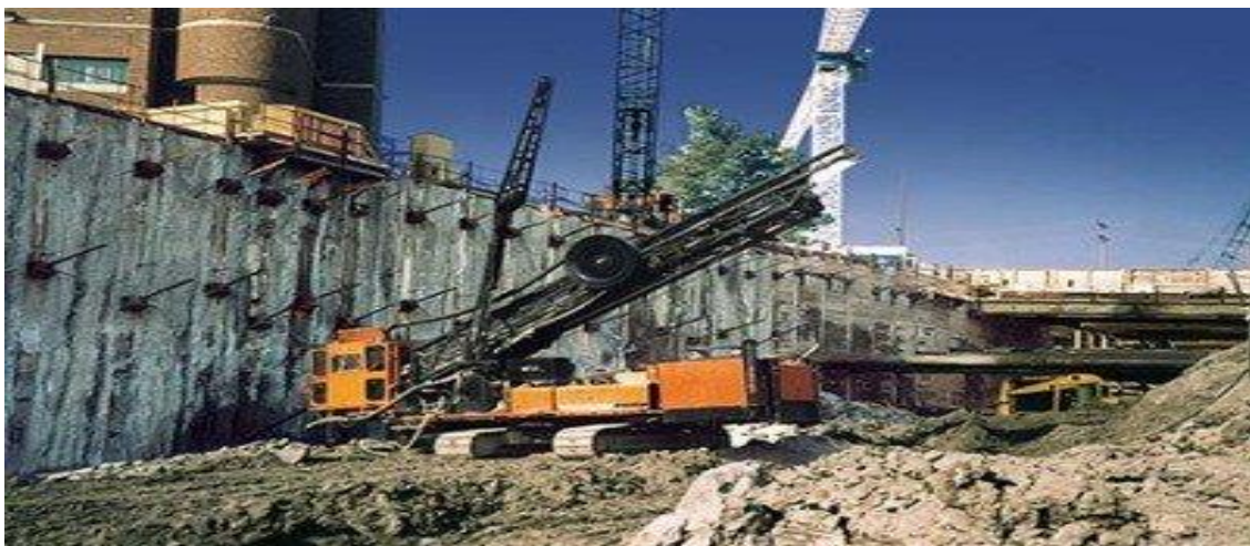
Fig. 3 – Excavation using Anchor Method
