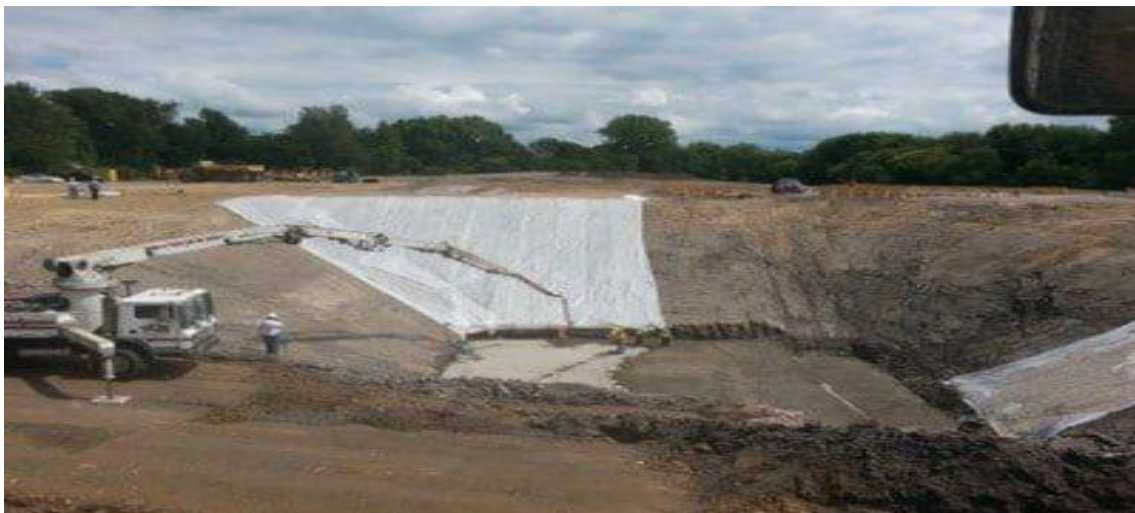
Fig.1 – Sloped open cut.
