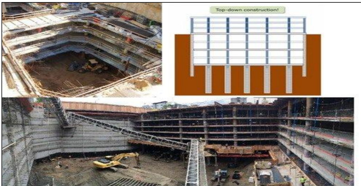
Fig. 5- Top-Down Excavation using slabs
