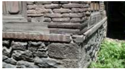
Fig.4: Shows the iron braces placed on corners, which increase the seismic resistance of buildings.
