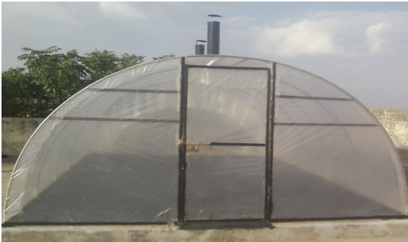
Figure1.2: Front view of solar tunnel dryer at UCE, RTU, Kota
