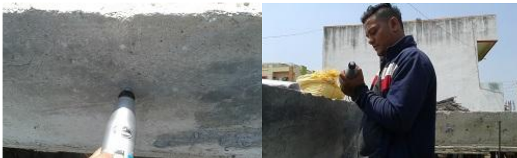
Fig.5 Rebound Hammer Test
