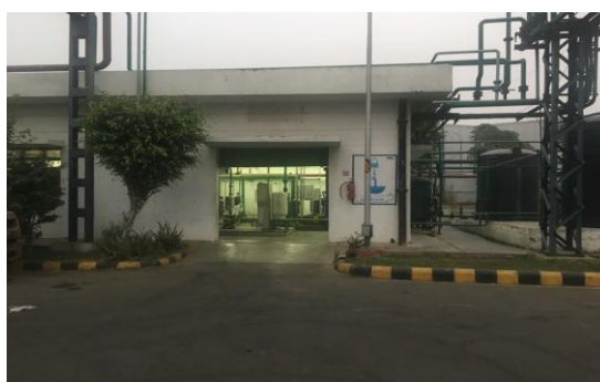
Image 4. Represent the control room for controlling the all process water waste treatment.
