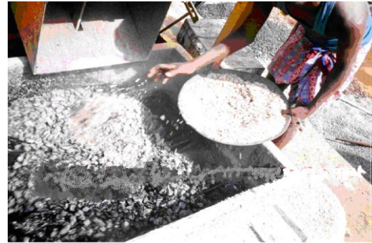
3.2 Shredded plastic waste is added
