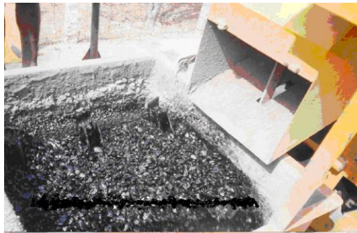
3.1 Hot bitumen is added
