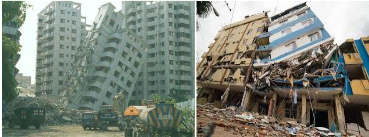
Figure 2: structures damaged due to earthquakes
