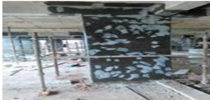
Fig.2:Application of epoxy putty
