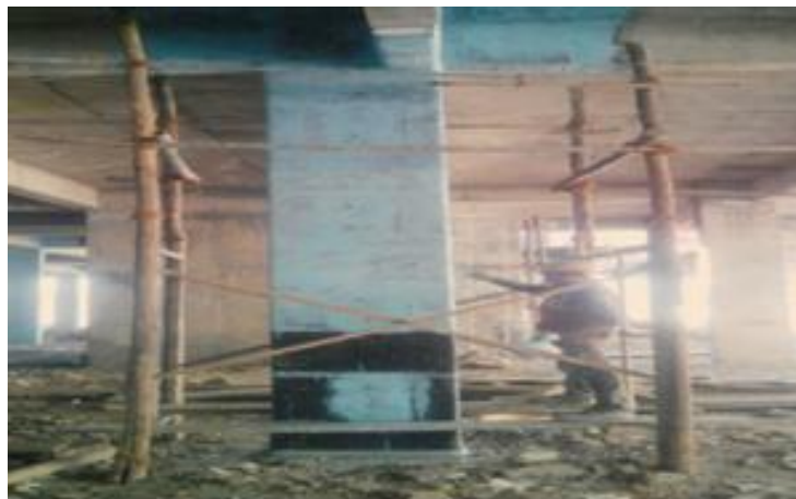
Fig.1: Primer Coating on column
