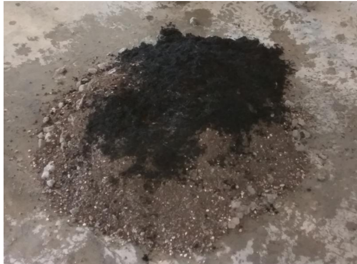
Fig.2.3 Mixing of shredded rubber in concrete
