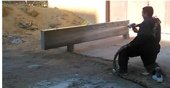
Fig (6): Spray of Polyurea
