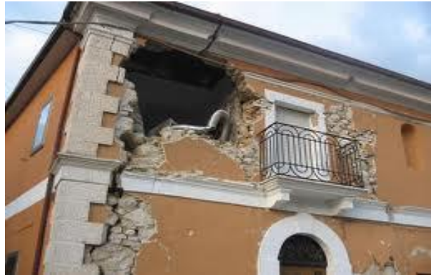
Fig. 1 Earthquake Struck Non-Engineered Building [5]
